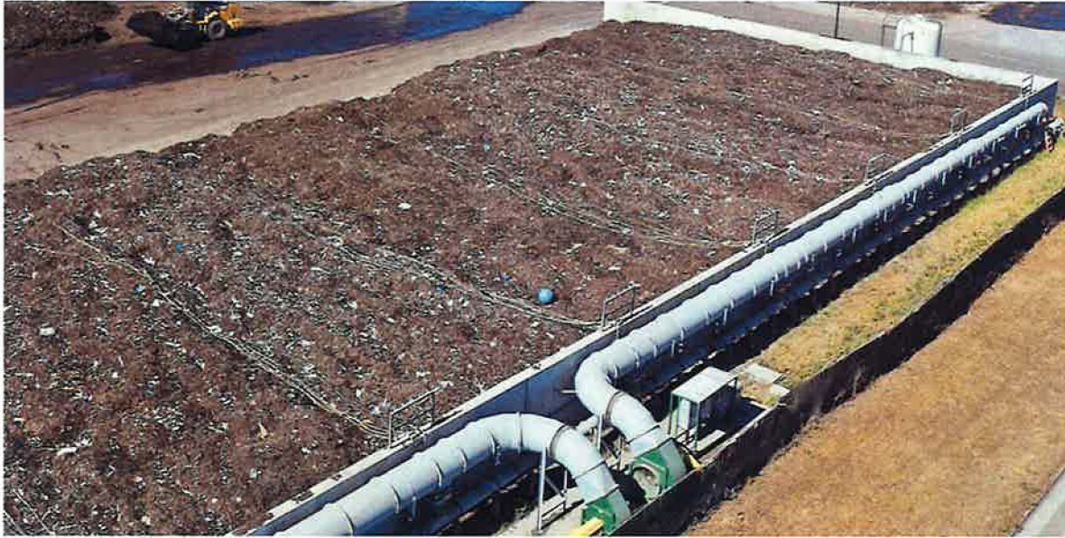
Figure 5 - positively aerated ASP with mass-bed configuration and concrete pushwall
