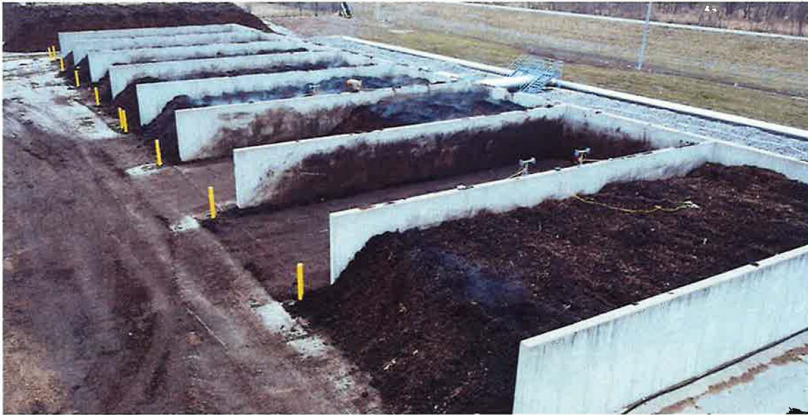
Figure 4 - Biosolids compost facility with concrete bunker walls, trench style floors and biofilter
