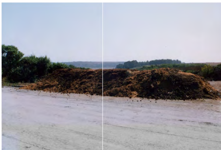
An impermeable surface, graded to control runoff.
