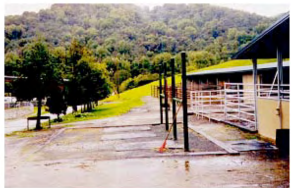
This horse wash area drains into a grass filter strip (along the row of trees). The filter strip traps sediment, horse manure and other contaminants.
