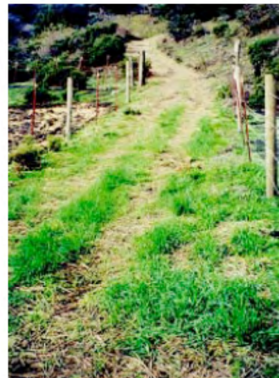
Roads not used in the winter can be “put to bed” for the season. This road has been seeded and will not be used again until the spring. Roads should be properly graded, seeded and mulched, to help prevent erosion. Seeding should occur before October 15 to ensure adequate growth before the winter rains.
