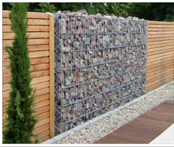
6' GABION / WOOD FENCE WITH STEEL SUPPORT POST.
