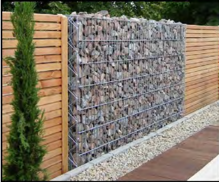
Figure 8 - Proposed 6' Gabion/Wood Fence
